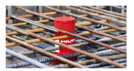
"Hilti cast-in devices create the opening for the pipes to go through and at the same time offer an integrated firestopping system. This product is so efficient and easy to install. We have installed 5,000 pieces and we had zero failures."
