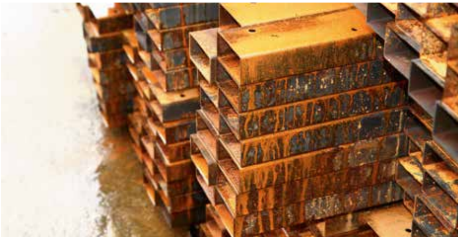
Fig. 4: Corrosion of steel components.
