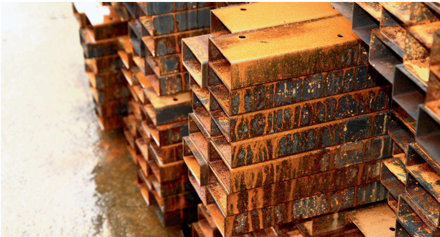
Fig. 4: Corrosion of steel components.
